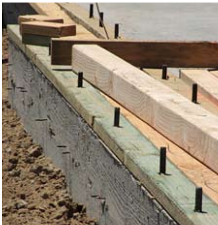
No more pre-drilling sill plates to accommodate cast-in-place bolts
