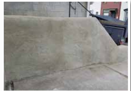
The degraded wall has been given a new life cycle and a brand new appearance.
