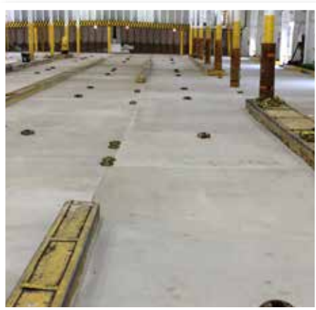
Existing surface cleaned, prepared and primed with Elephant Armor® Overlay Primer.
