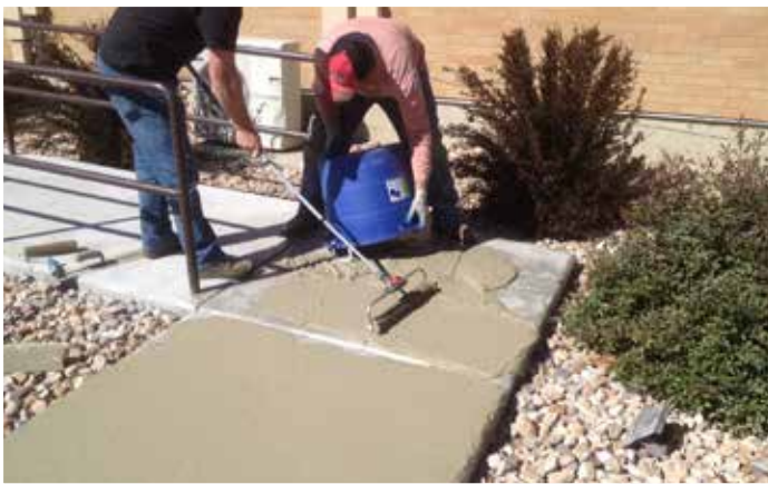
Elephant Armor® rolled over pre-primed surface using 1/4" gauge.
