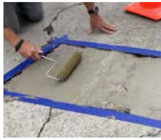
Cracks are pre-filled with Elephant Armor®.
