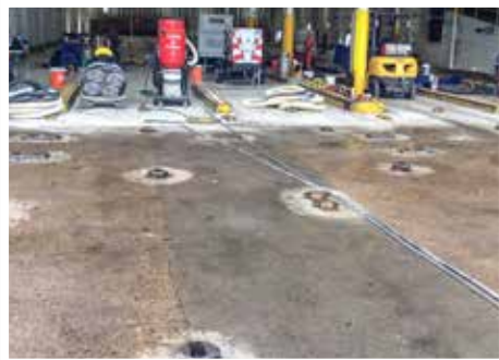
Existing surface cleaned, prepared and primed with Elephant Armor® Overlay Primer.
