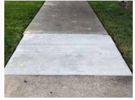
Finished repair with a new lifetime of service. Open for use within two hours of placement.
