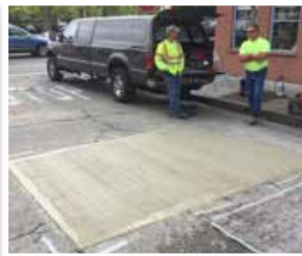
Repair completed with a broom finish.
