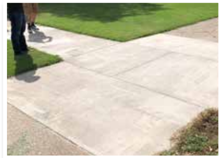
Finished project opened to foot traffic within an hour of completion.
