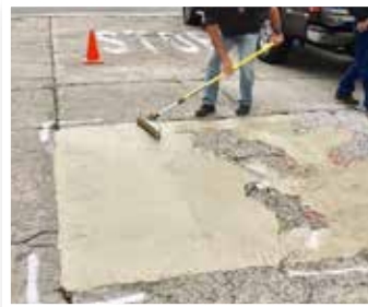
Elephant Armor® being applied using a roller.
