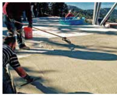
Elephant Armor® applied with rollers and trowels.
