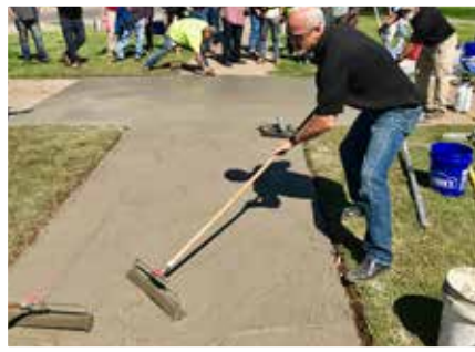
Applying Elephant Armor® using GST's specialty rollers and tools. (see page 11)
