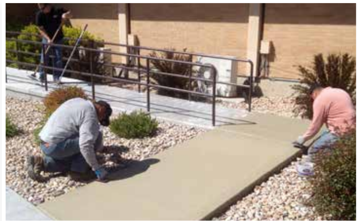
Overlay being finished using traditional finishing tools.
